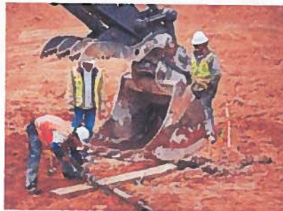
Steve Herrera Judicial Complex - Site environmental clean-up
