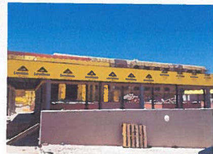
Steve Herrera Judicial Complex - Construction progress
