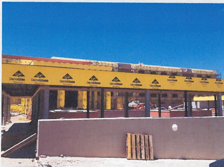
Steve Herrera Judicial Court Complex Construction – Front View
