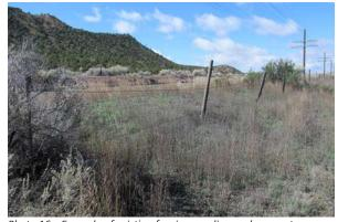
Photo 16. Example of existing fencing needing replacement.
